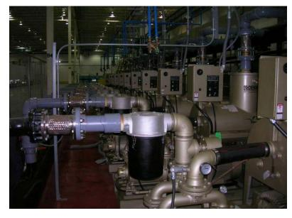
The operation of the individual vacuum systems is identical to the simplex Vmax. The entire unit is controlled by the use of vacuum switches, PLC logic, or the DEKKER controller. The operation of the system can be varied through the use of the HOA (Hand / Off / Auto) switch on the control panel.
