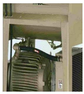
On air cooled Vmax systems, the seal fluid travels through the heat exchanger and is cooled by a motor-mounted fan. Standard air flow up to late 2001 was outside in (pull fan). Standard air flow after late 2001 is inside out (push fan).
