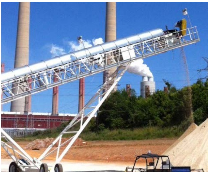
Flue Gas Desulfurization (FGD) Belt Filter Conveyor
