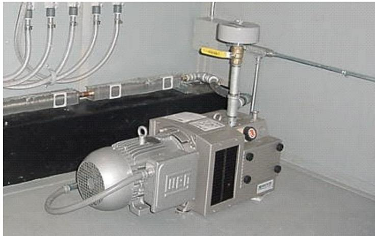
Figure 5: Rotary vane compressor package
