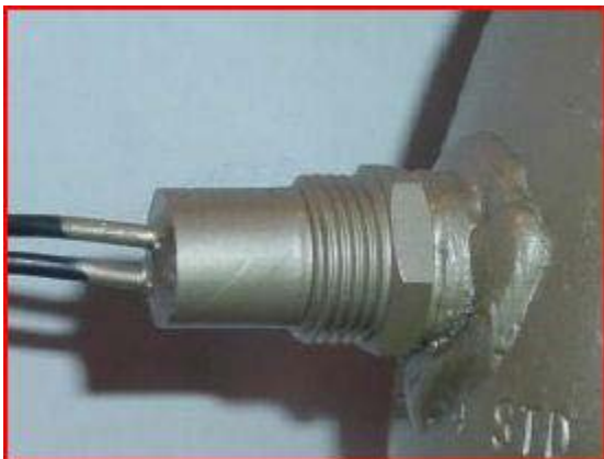
Temperature switch inserted into the pump discharge manifold.
